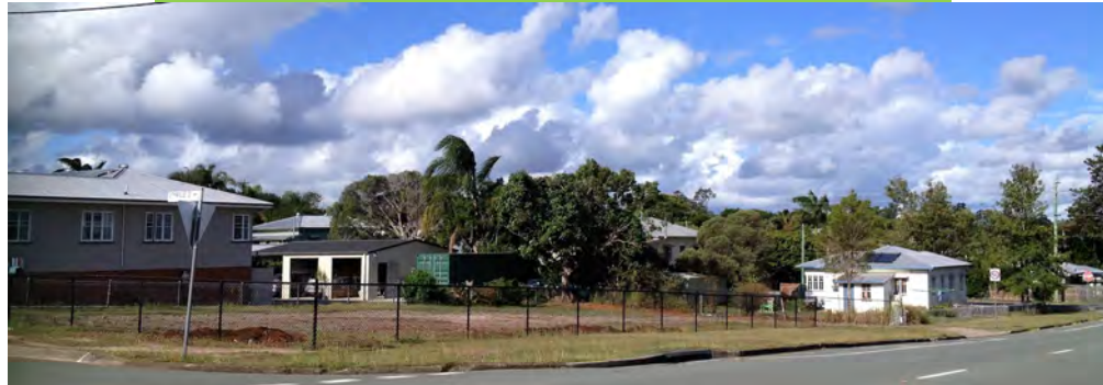
The empty Parish Office block, soon to contain the Presbytery
