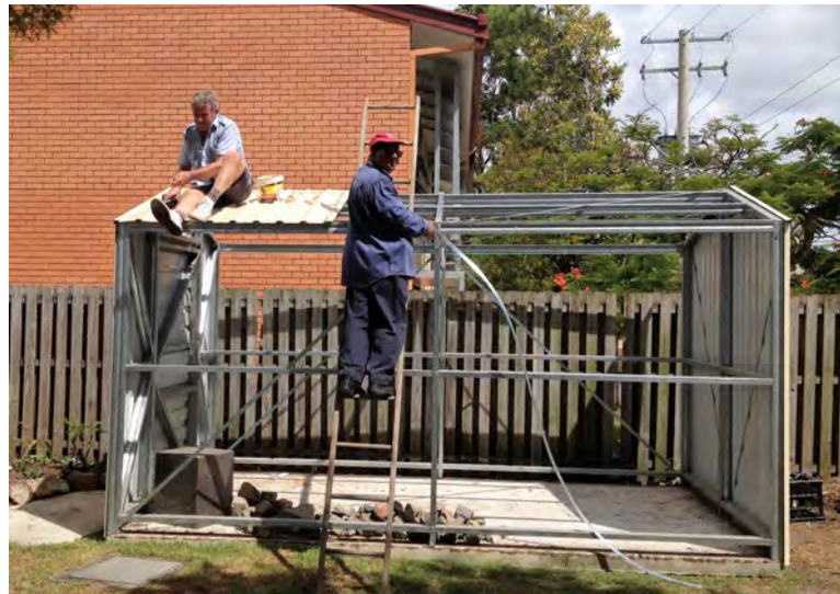
John and George making room for the garage / storage shed
