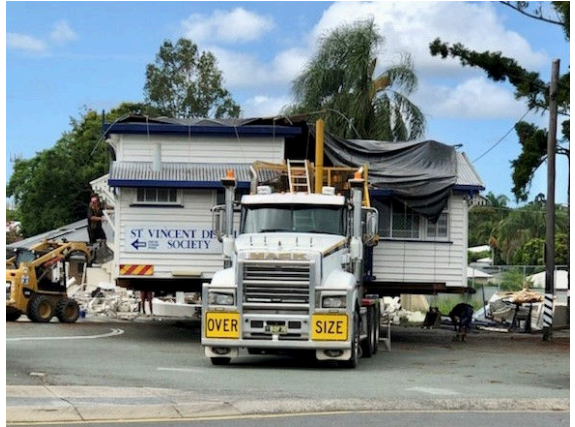
St Vinnies building being transported to its new home
